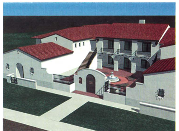
The two-story residence hall will provide living space for 106 men.
