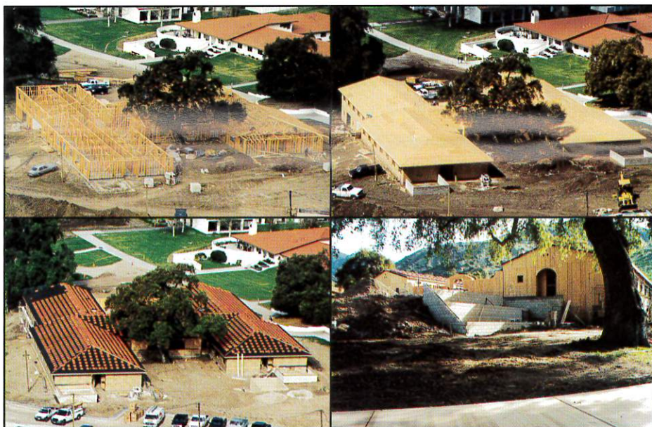
Upper left: Framing Lower left: Tile roofing
